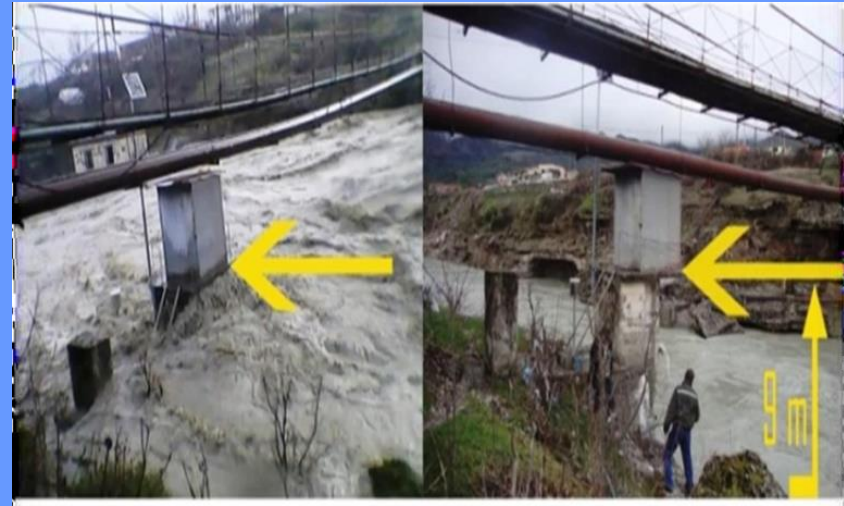
Damages in bridges, Vjosa river basin
