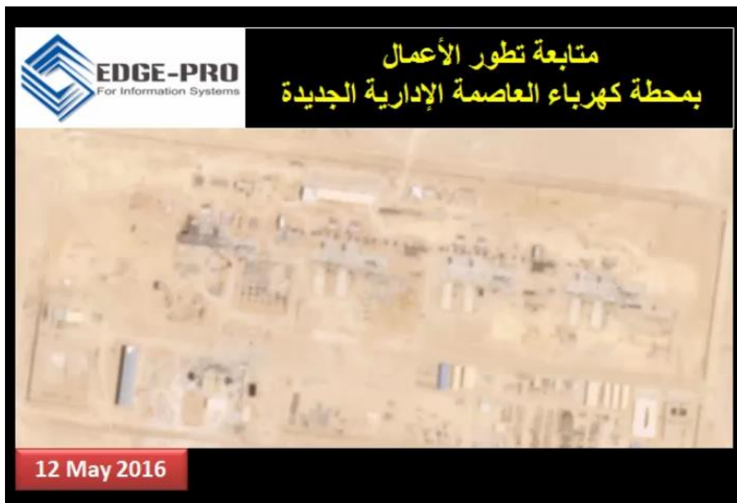
New Capital Power Station
